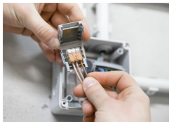
Place the wired connector in the Gelbox.
